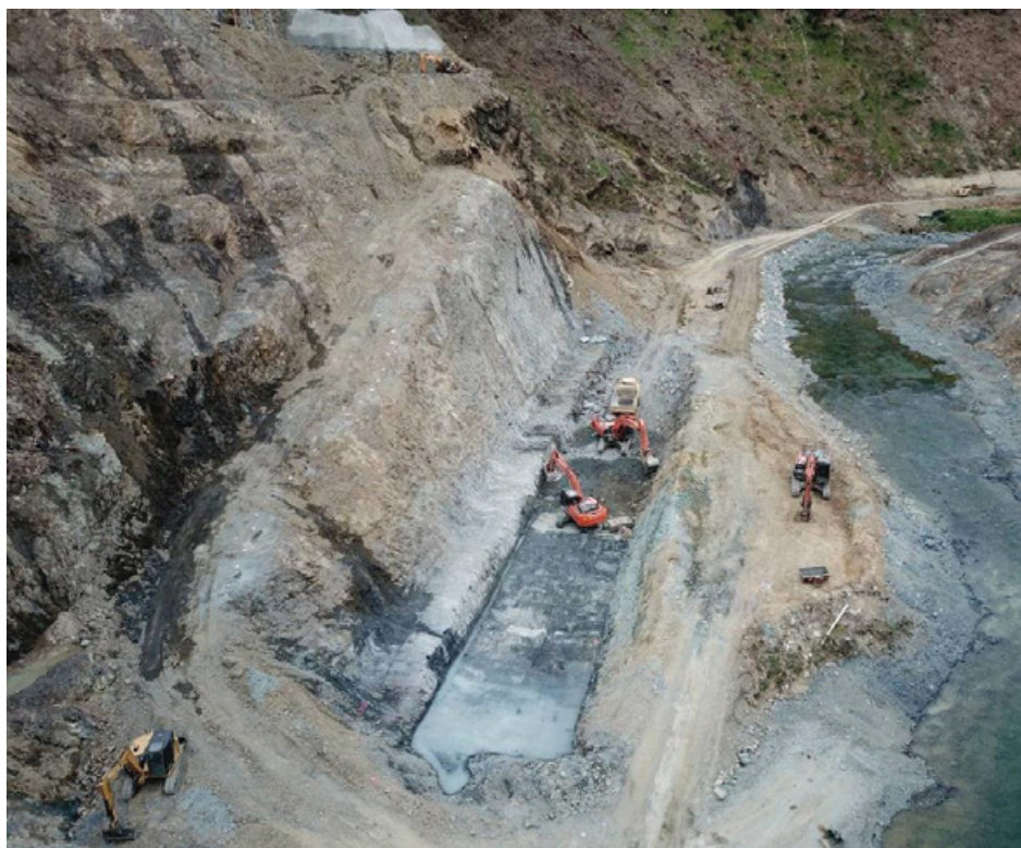
IMAGE: Waimea Dam under construction. Lee Valley, Nelson
